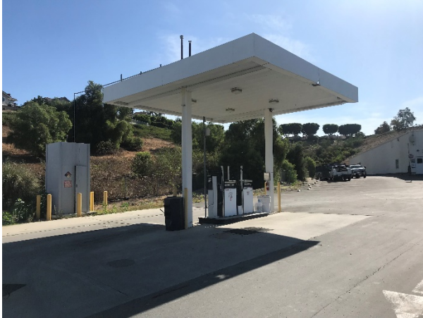
Existing Fueling Station
