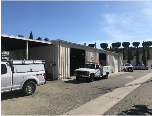
Existing Fleet Services Building
