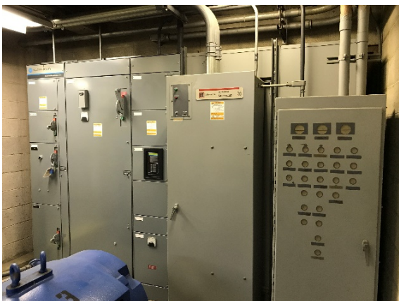
Existing Electrical Equipment to be Replaced at Pacific Island Dr. No. 3 Pump Station
