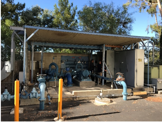
La Paz Pump Station Site
