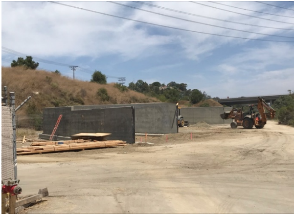
Newly Poured Material Bins in North Yard
