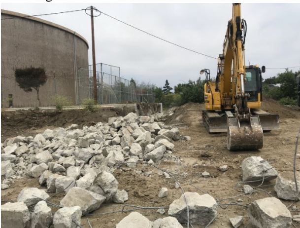
Demolition of Existing Wall in South Yard
