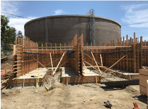
Forming New Material Bins in South Yard
