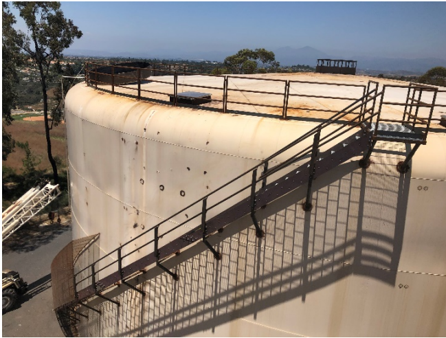
Bear Brand Reservoir Exterior to be Recoated
