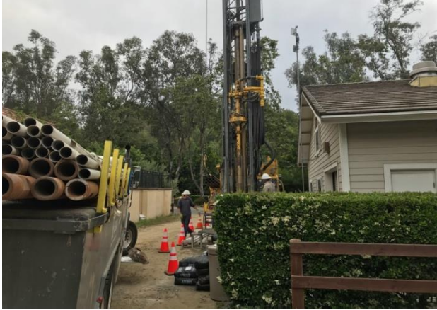
Anode Drilling at Bridlewood Pump Station
