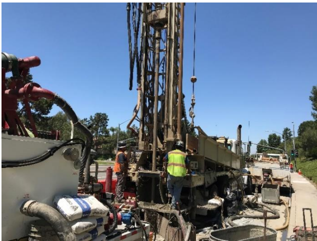
Anode Drilling at San Rafael and Oso Parkway
