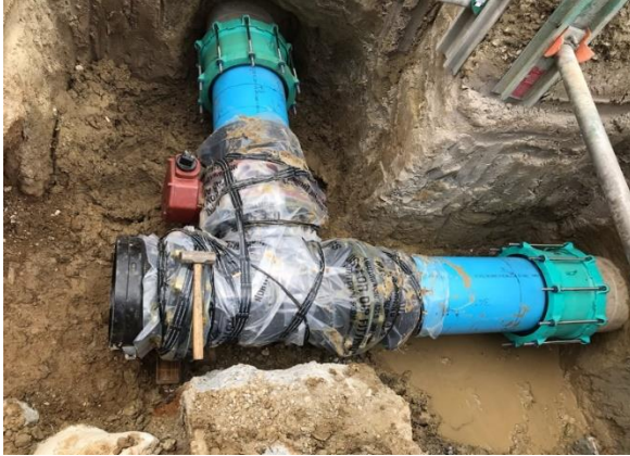
Installation of New Valves and Tee at Isle Vista Way
