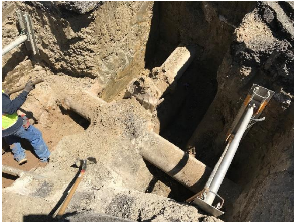
Excavation for Valve Replacement at Tropea Way and Marina Hills
