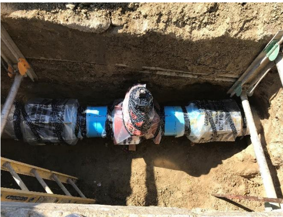
New Valve at Marina Hills and Golden Lantern
