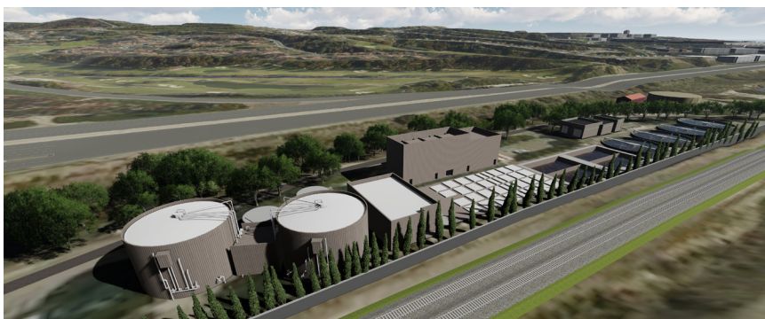
Figure 1. 3-D Aerial View of Plant 3A
