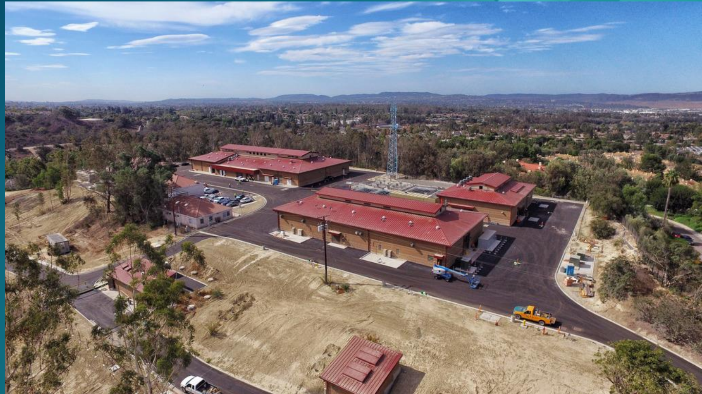
Image of Baker Water Treatment Plant
