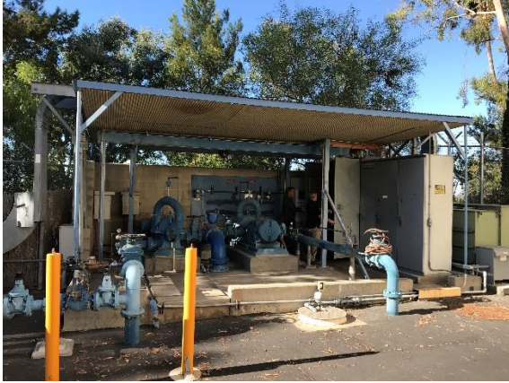
La Paz Pump Station Site
