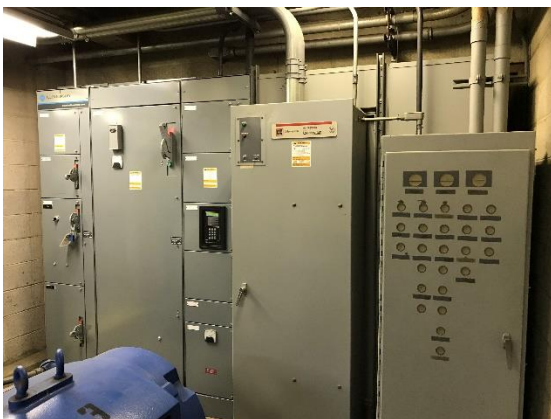
Existing Load Bank to be Replaced at Highlands Pump Station
