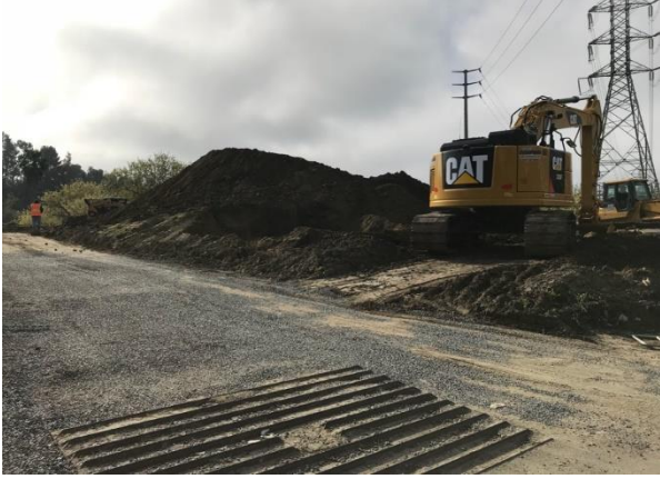
Grading of South Yard
