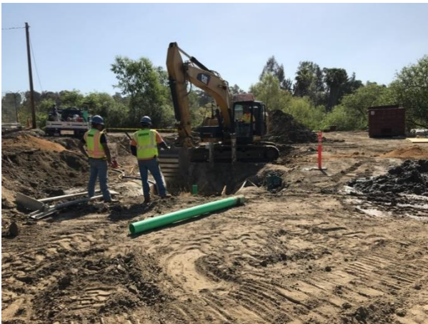
Excavation for Drain Improvements
