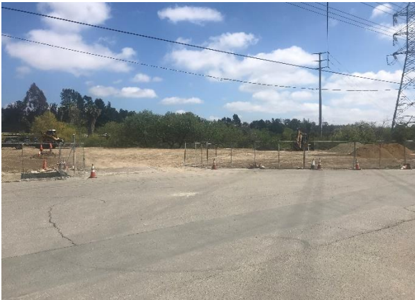
Completed South Yard Grading
