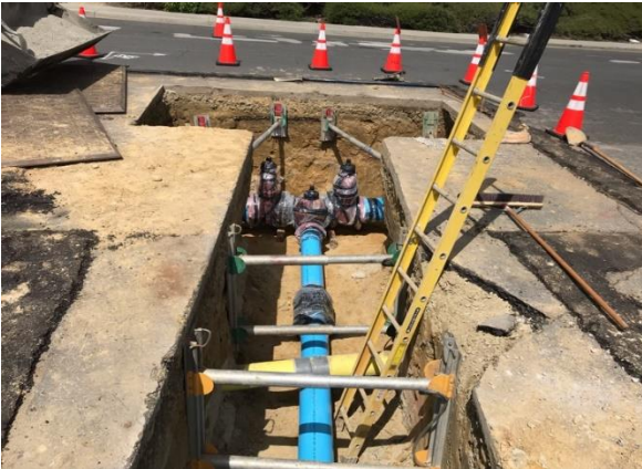
Replacement of Three Valves and Connection to Mainline at Highlands and Niguel Rd.
