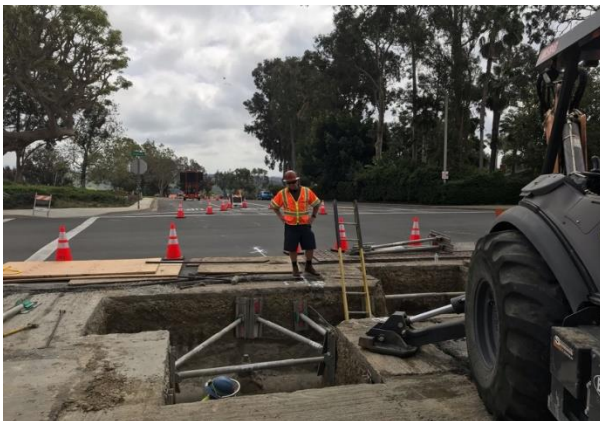
Excavation for New Valves at Isle Vista and Ocean Way
