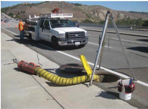
Typical Required Manway Entry
