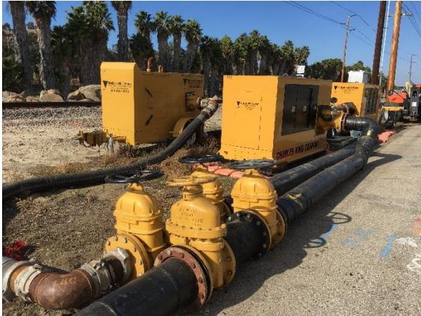
Oso-Trabuco Bypass Set-up
