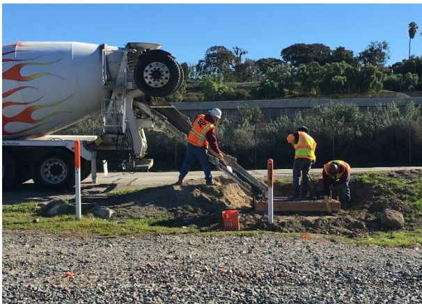
Crews Pour New Pad at Existing Manhole
