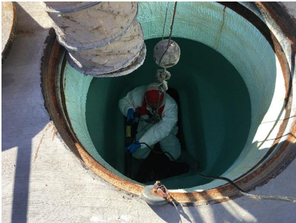
Re-coating of Existing Manhole
