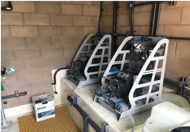
Newly Installed Chemical Dosing Pumps
