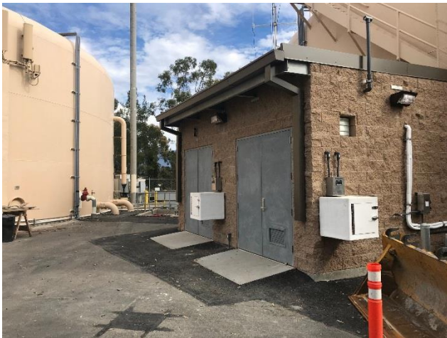
Seville Reservoir New RMS Facility
