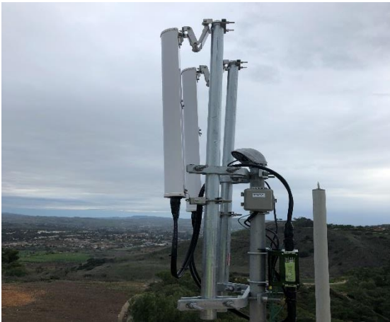
Highlands Pump Station Antenna Install
