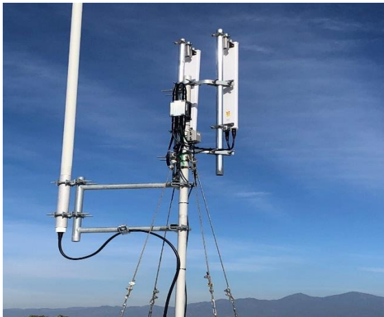
Newly Installed AMI System
