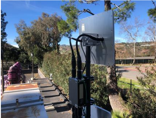
Rancho Reservoir Antenna Install
