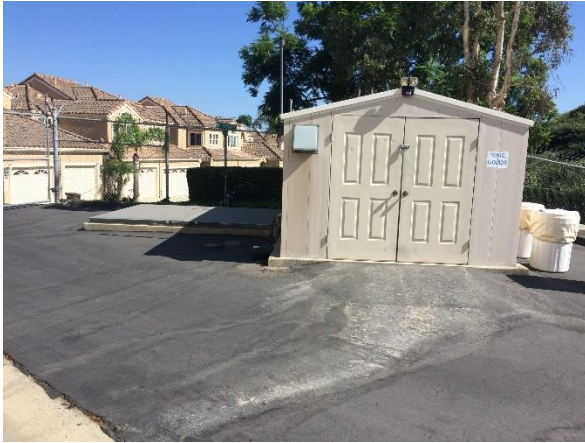
Existing Chlortec Building at Highlands Reservoir
