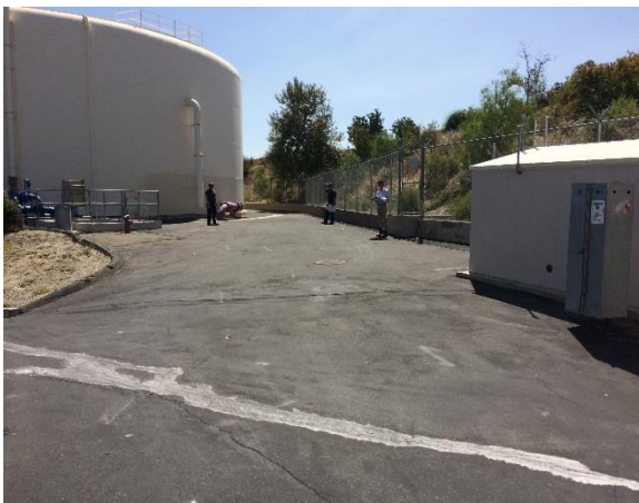
Site Visit and existing Chlortec Building at Moulton Peak Reservoir
