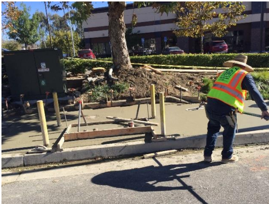
La Paz Underground Exterior Concrete Work
