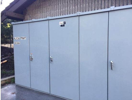
Newly Installed Electrical Cabinets at Regional Lift
