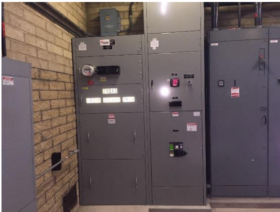
New Main Switchboard at Crown Point Pump Station
