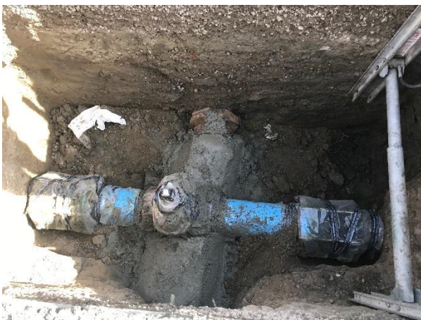
New Piping and Valve on Niguel Rd.
