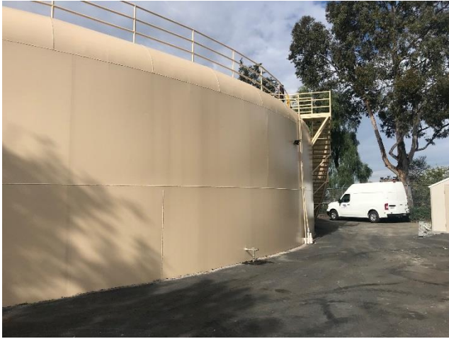
Completed Exterior Coating
