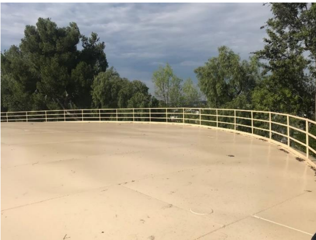
New Perimeter Roof Guard Railing
