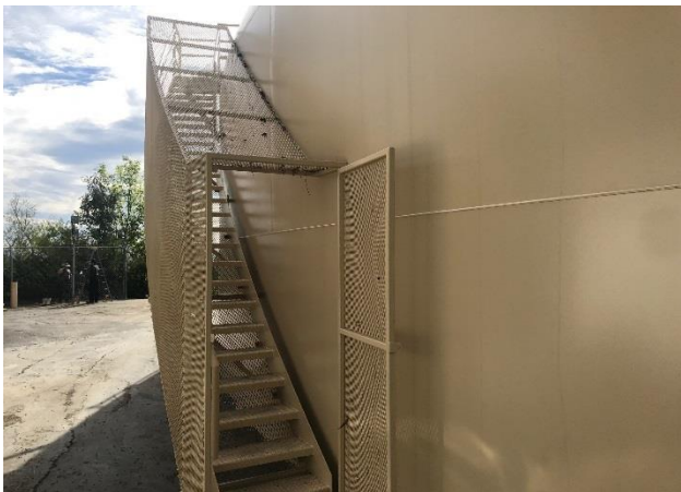
Newly Installed Spiral Staircase
