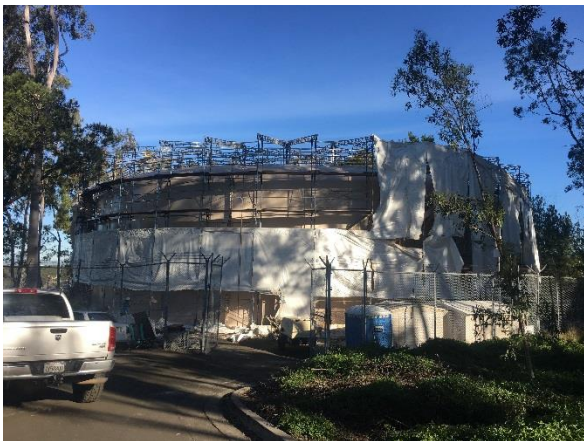
Removal of Exterior Containment Structure
