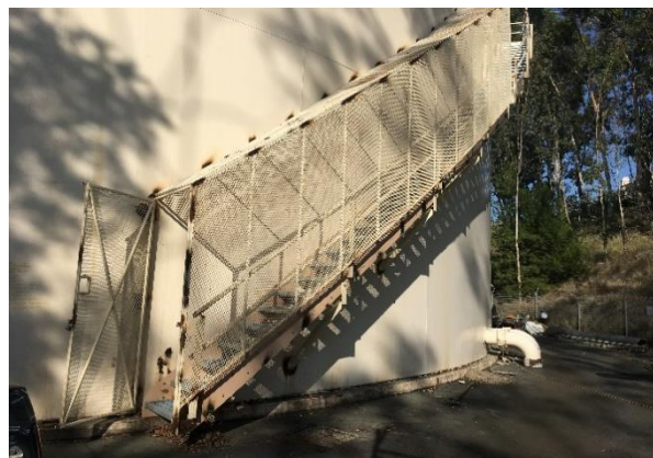
New Spiral Staircase
