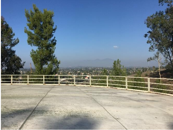
Newly Installed Handrails
