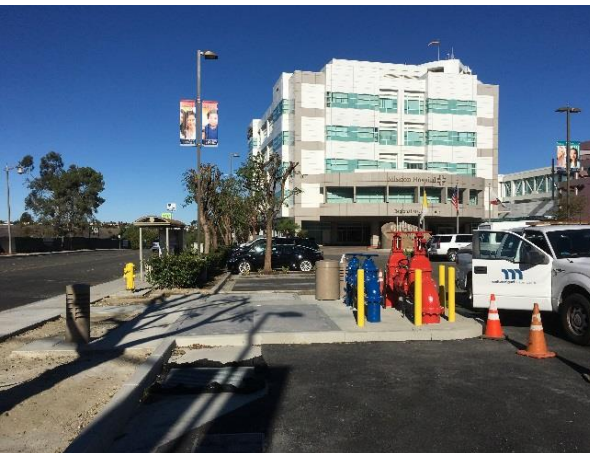
Completed Pressure Reducing Station
