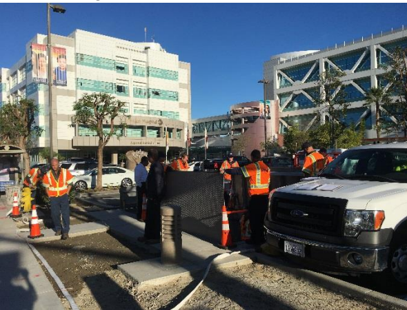
Start-up Testing with Mission Hospital Staff
