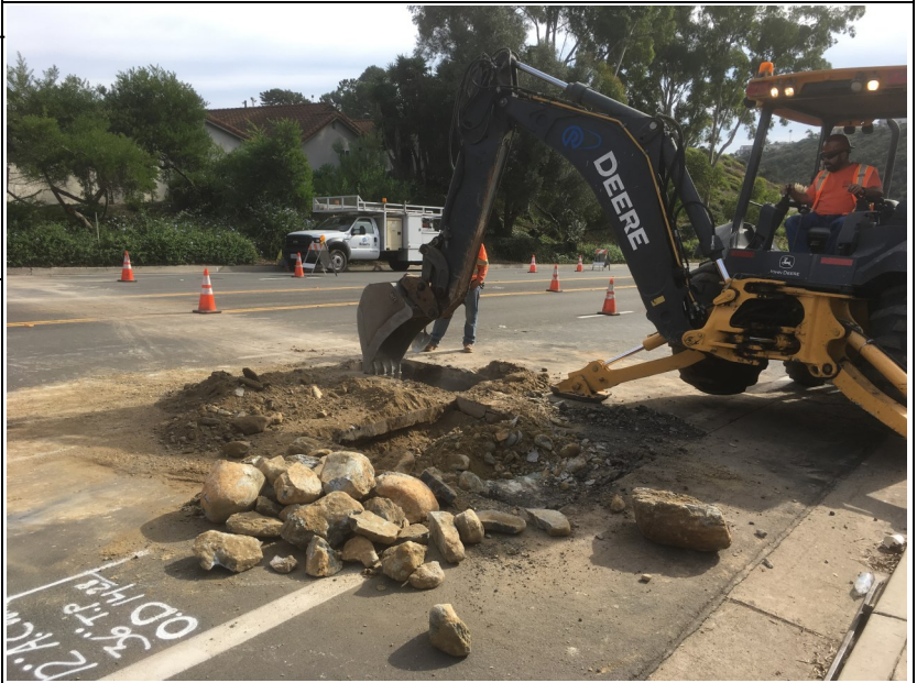
Preparation for Installation of new 8-inch Mainline
