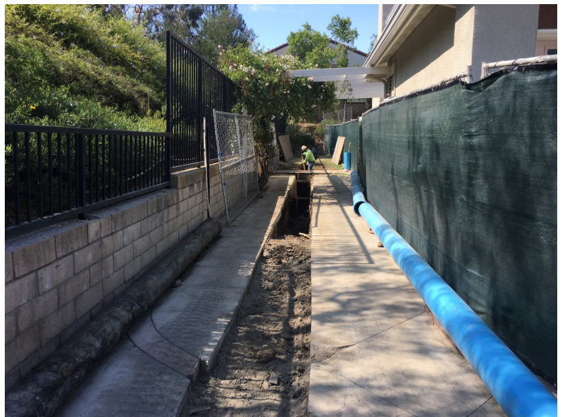
Installation of 8-inch Potable Easement Mainline
