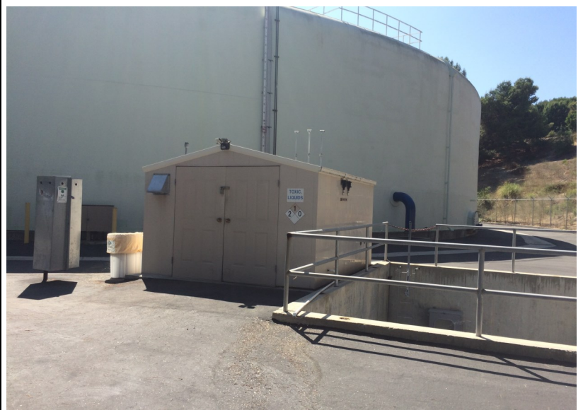
Existing Reservoir Management System (RMS) Building
