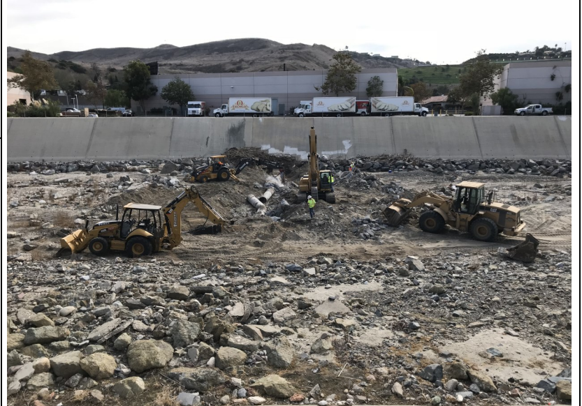
ETM Pipeline Removal
