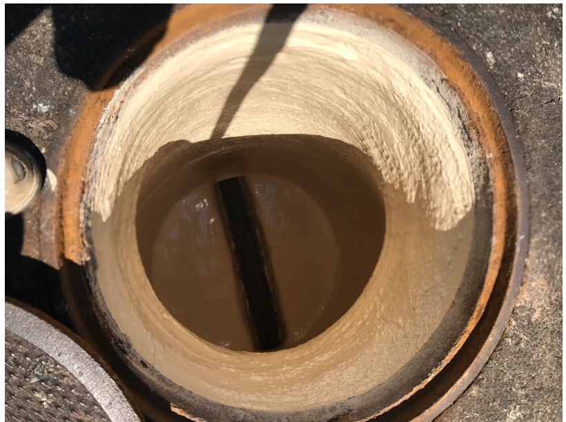
Rehabilitation of Manhole in Mission Viejo
