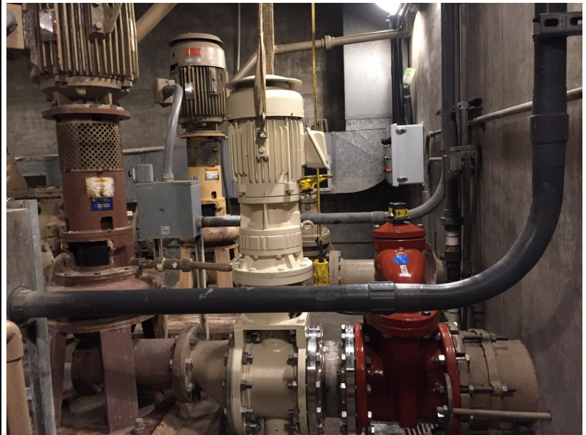
New Valve and Grinder
