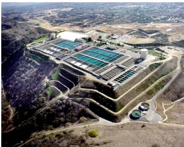
Diemer Filtration Plant
