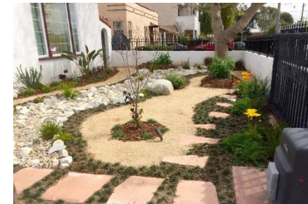
Contractor installs new landscape
