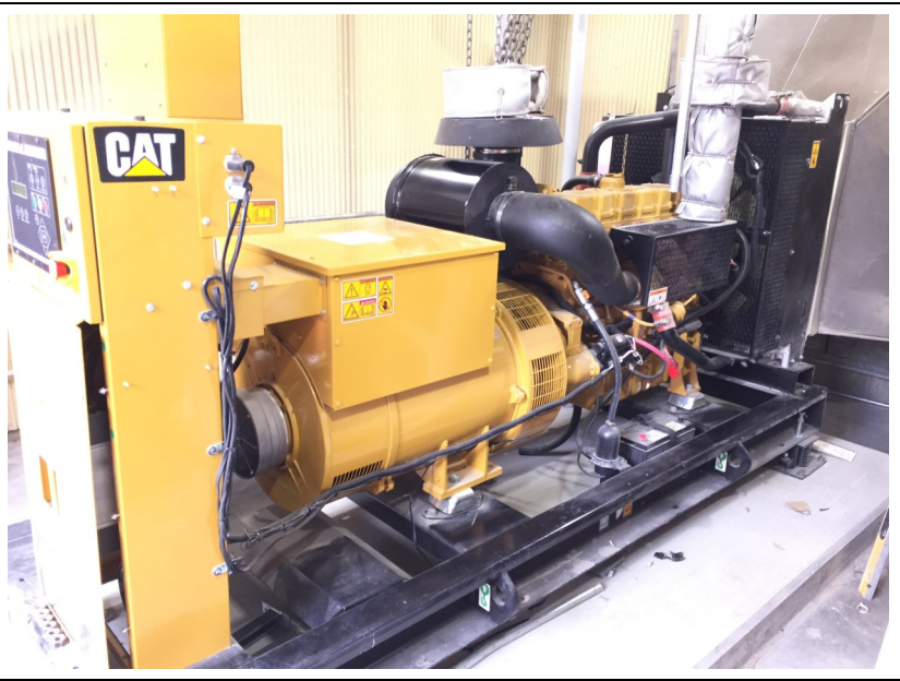
New Emergency Standby Generator
