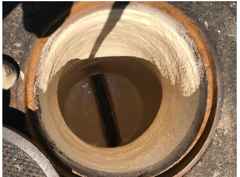
Rehabilitation of Manhole in Mission Viejo
