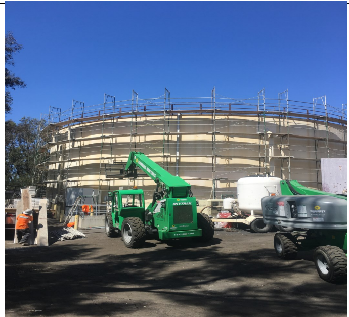
Crown Valley Reservoir 2 Exterior Coating Prep
