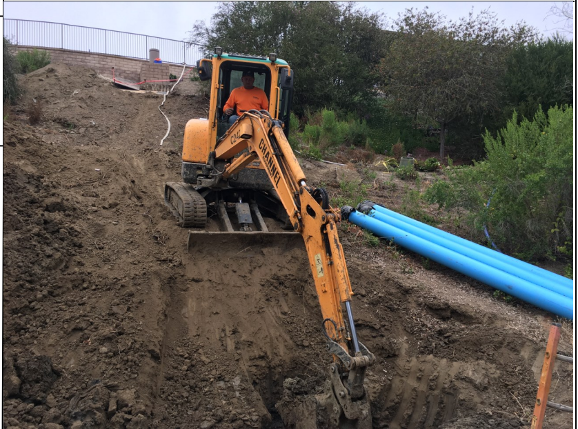
Exposing Existing Easement Line for Replacement
