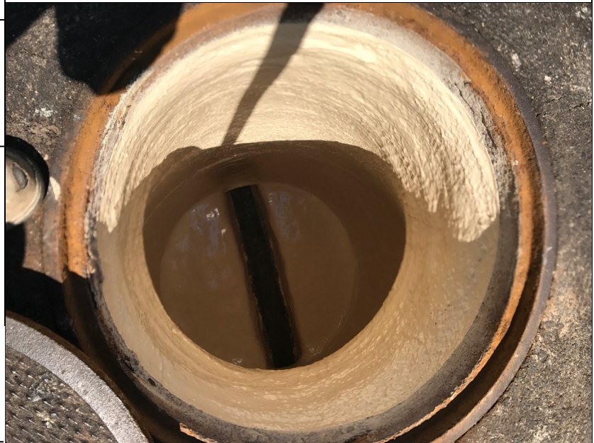
Rehabilitation of Manhole in Mission Viejo
