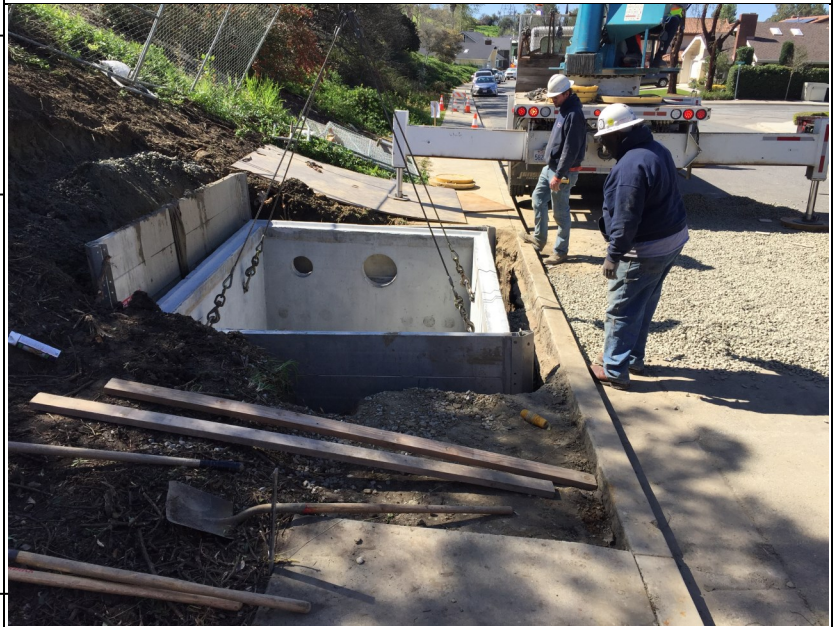
Installation of New Pressure Reducing Station Vault at Largo Dr.
