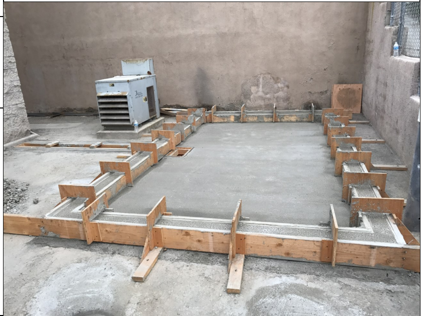
New Generator Pad at Del Avion Lift Station
