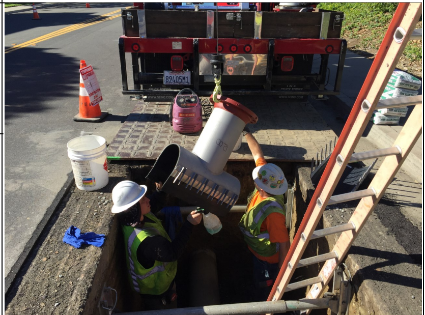
Installation of New Insertion Valve
