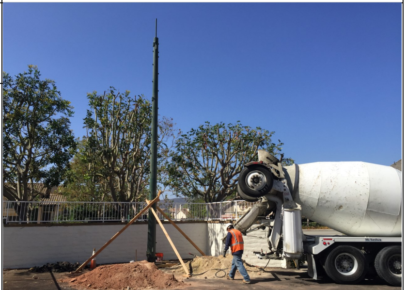
Monopole Installation at Audubon Lift Station
