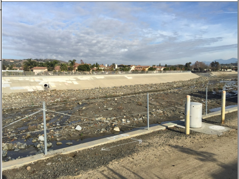
Completed Micro-Tunnel Project
