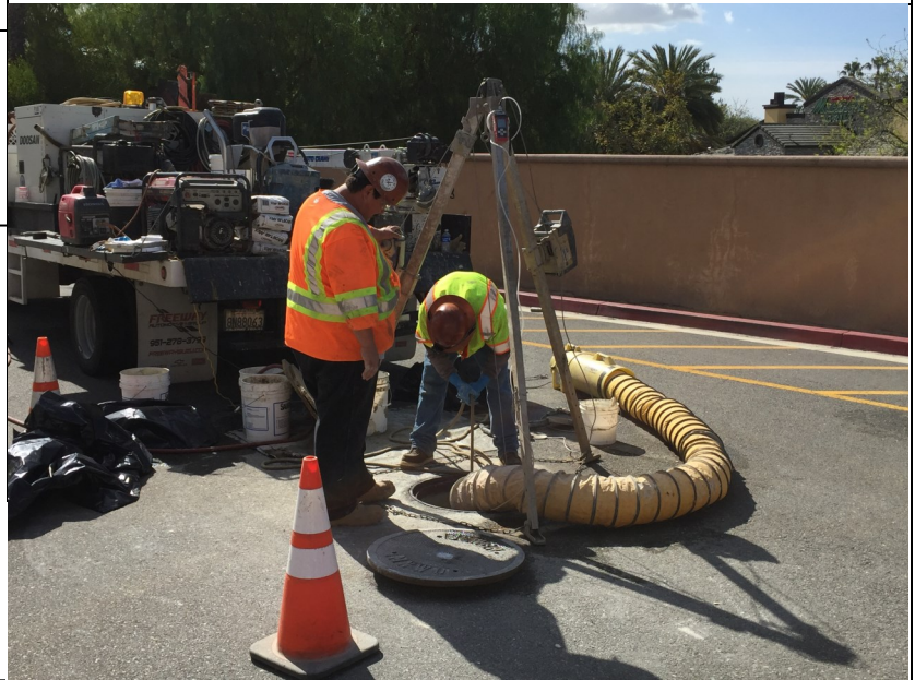
Rehabilitation of Manhole in Aliso Viejo
