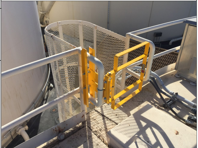
Newly Installed Swing Gate
