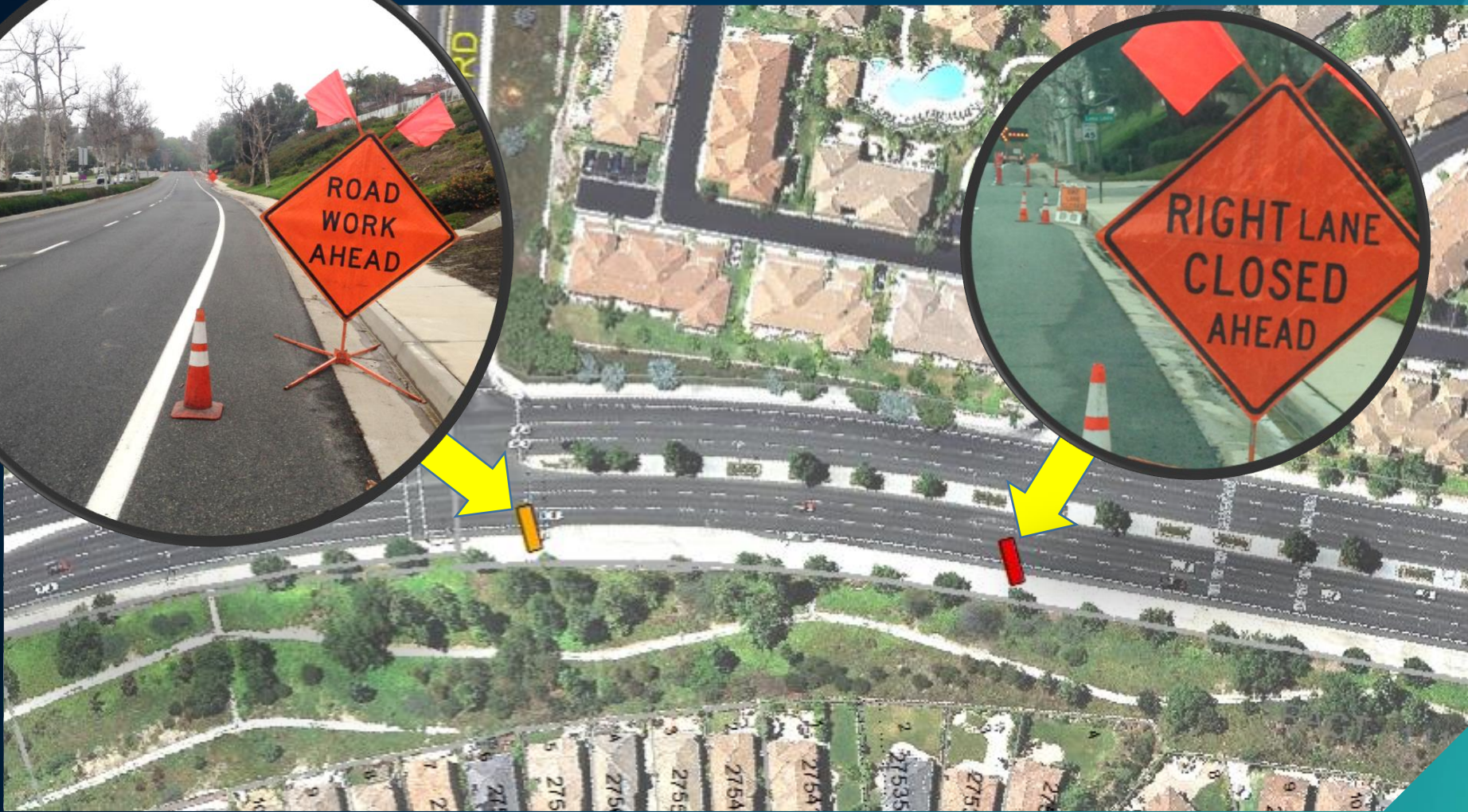
BEGINNING OF WORK AREA SIGNAGE — MOULTON PARKWAY / AVILA ROAD
