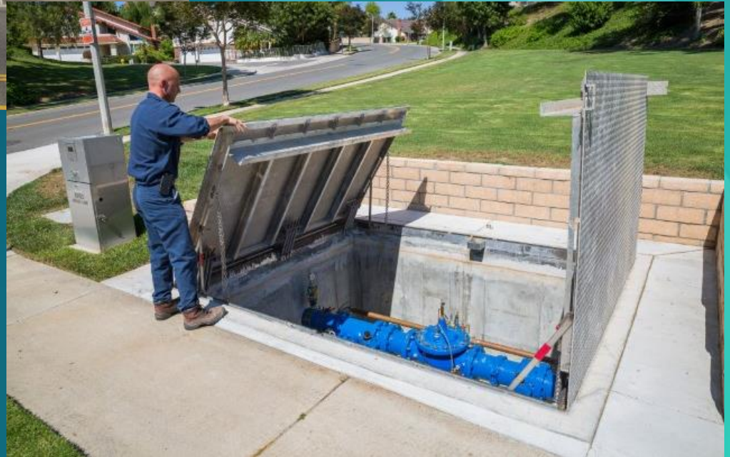
EXAMPLE OF SIMILAR PRESSURE REDUCING STATION
