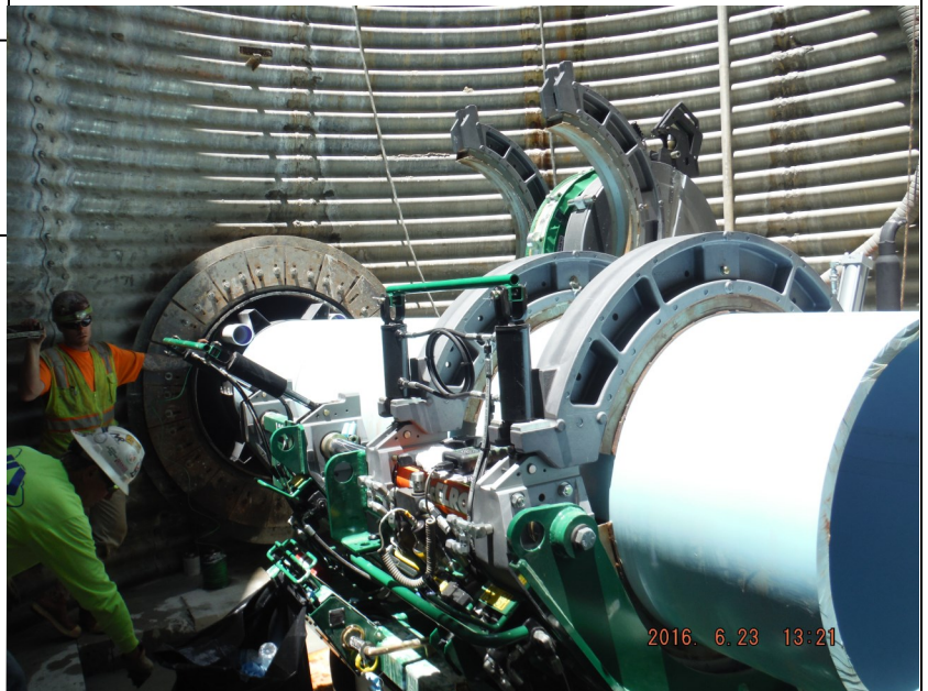
Installation of New 30" Sewer Main
