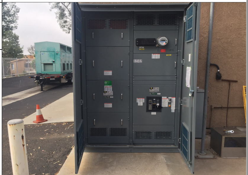
Lower Salada Lift Station New Main Breaker
