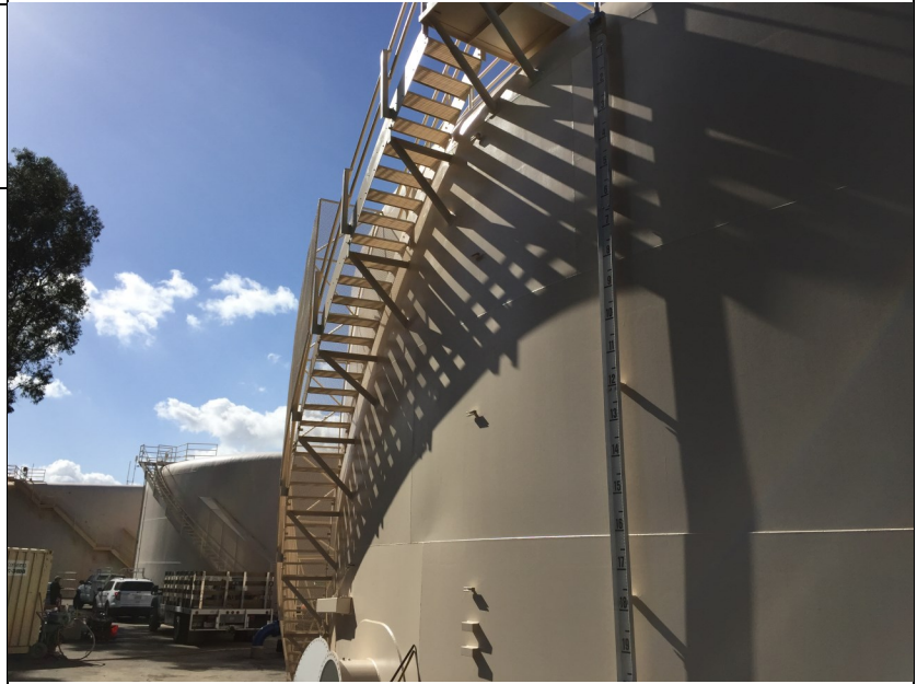
Mathis Recycled Reservoir New Staircase
