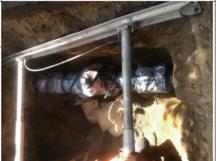
The Ranch at Nellie Gail Installation of Mainline
