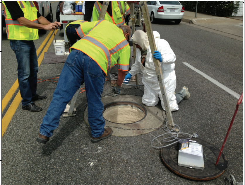
Manhole Locations in Mission Viejo Along Jeronimo and Alicia Parkway
