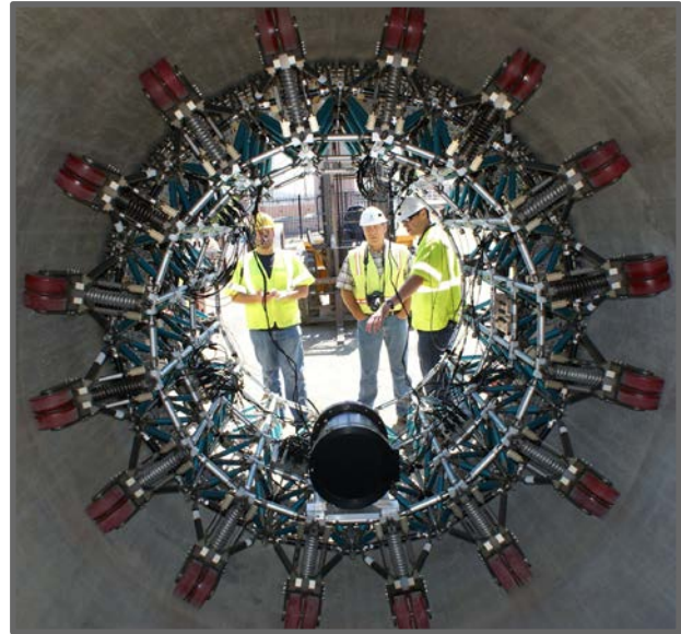
Figure 3: 96-inch MFL Tool used during inspection of Pipeline 4
