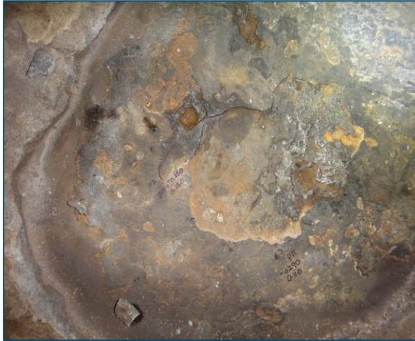
Figure 11: Wall Loss of a Steel Pipe
