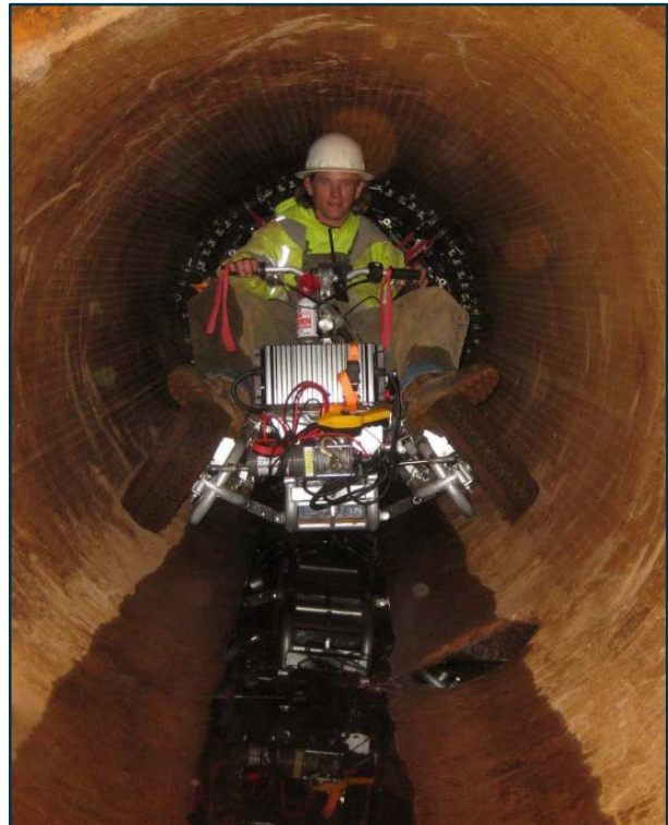
Figure 7: MFL inspection of 58" Pipeline
