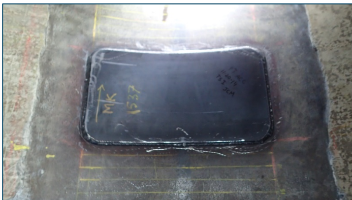
Figure 16: Welded steel patch repair on San Diego County Water Authority's Pipeline 3
