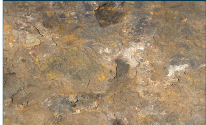
Figure 5: Corrosion pitting on the exterior of this pipe was consistent with MFL inspection data.
