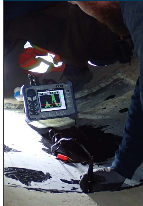
Figure 15: UT Verification of San Diego County Water Authority's Pipeline 3
