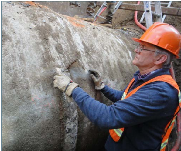
Figure 6: Exterior inspection of Pipeline 3
