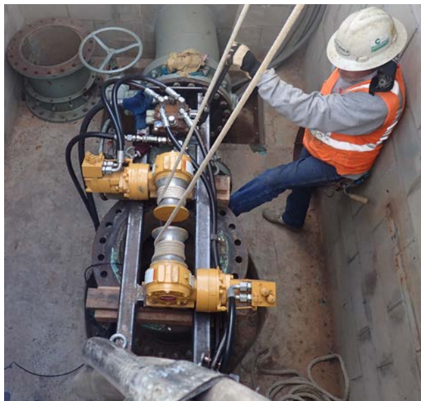
Figure 4: Winching of MFL Tool during the inspection of Pipeline 3
