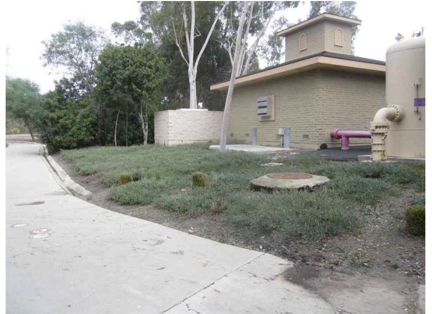
Site No. 8, Crown Point Pump Station
