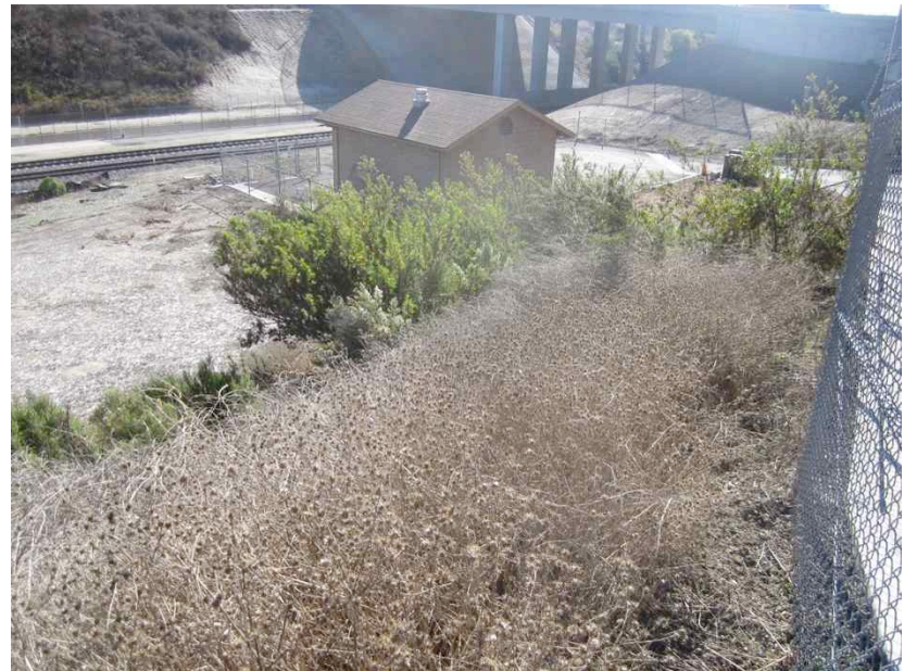
Site No. 4, Cabot Road Takeout
