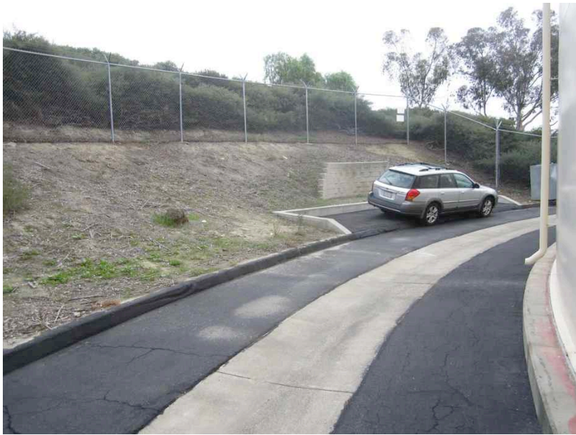
Site No. 13, Rancho Reservoir
