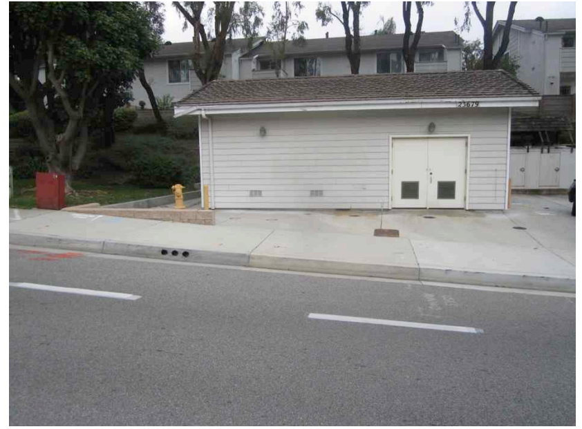
Site No. 10, Big Niguel Pump Station
