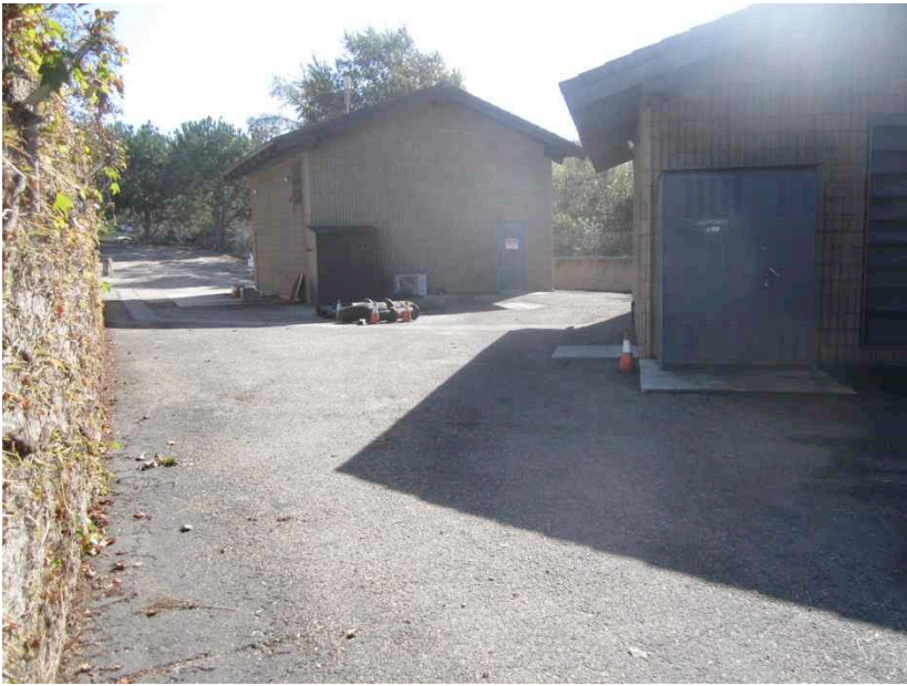
Site No. 1, Aliso Creek Lift Station
