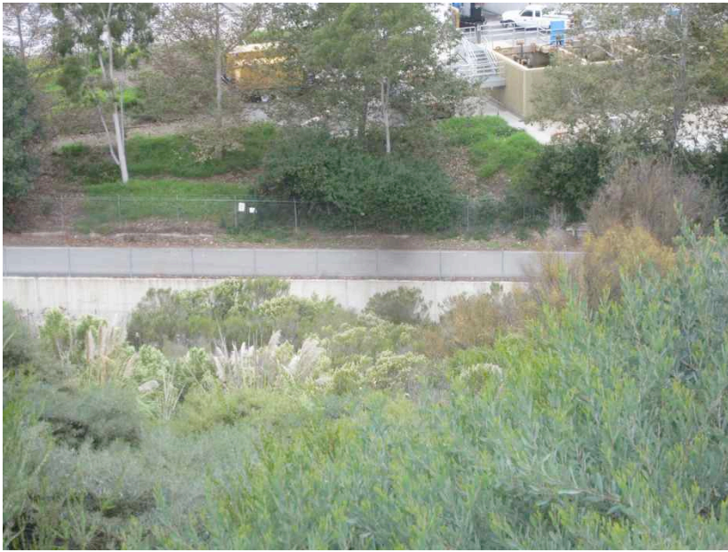
Site No. 9, AWMA2 Treatment Facility
